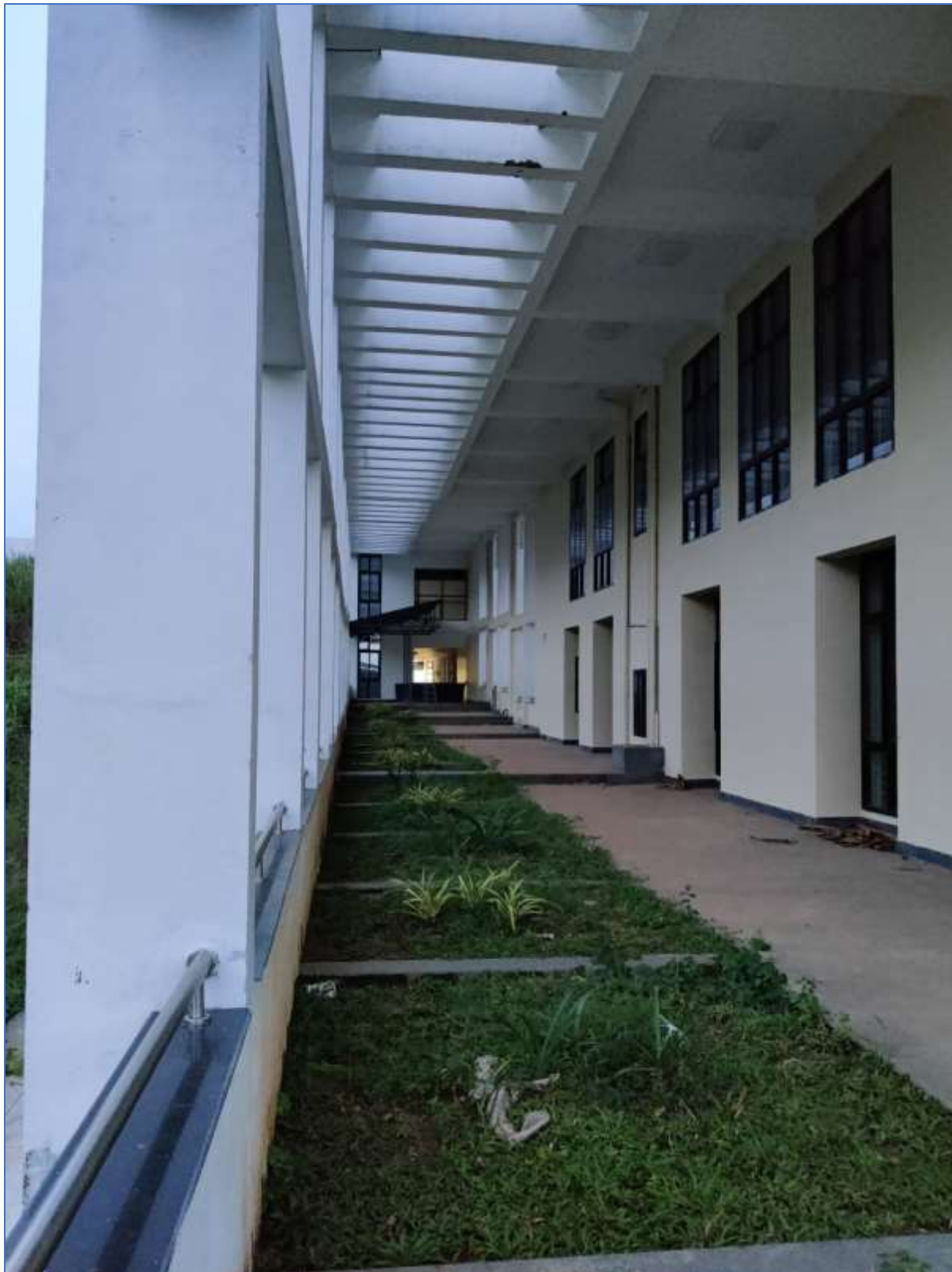
Passage between Academic Block 1 and Administrative Block
