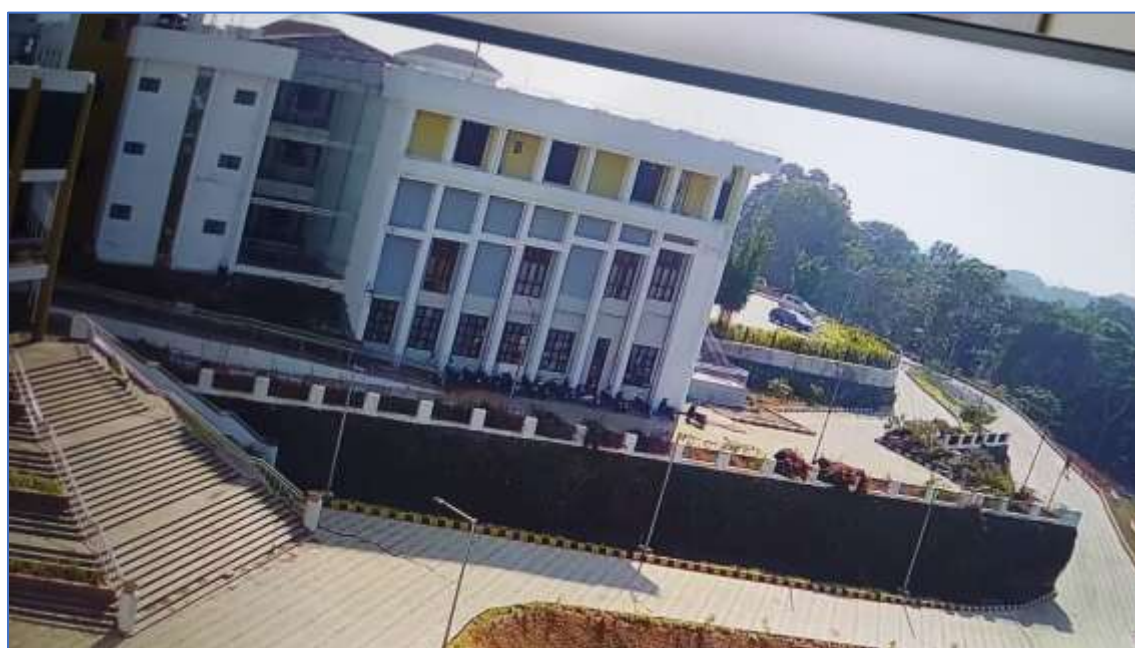
Entrance of Academic Block 2 and Administrative Block
