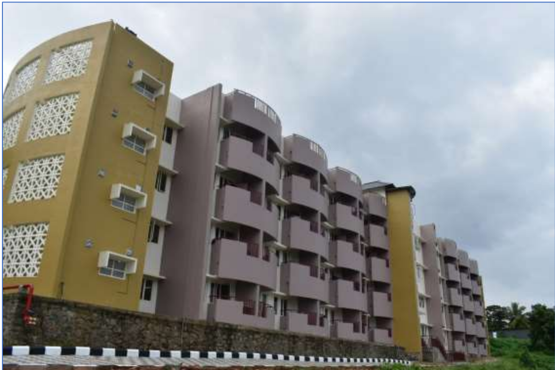
Hostel Number 3 (back view)
