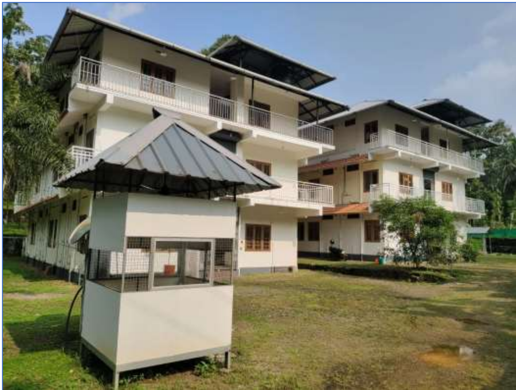
External Hostel – Block 1 & II – With Attached Bathrooms
