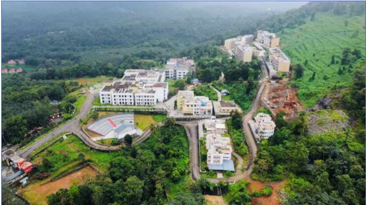
Arial View of entire IIIT Kottayam campus using Drone Camera (13 Nov 2022)
