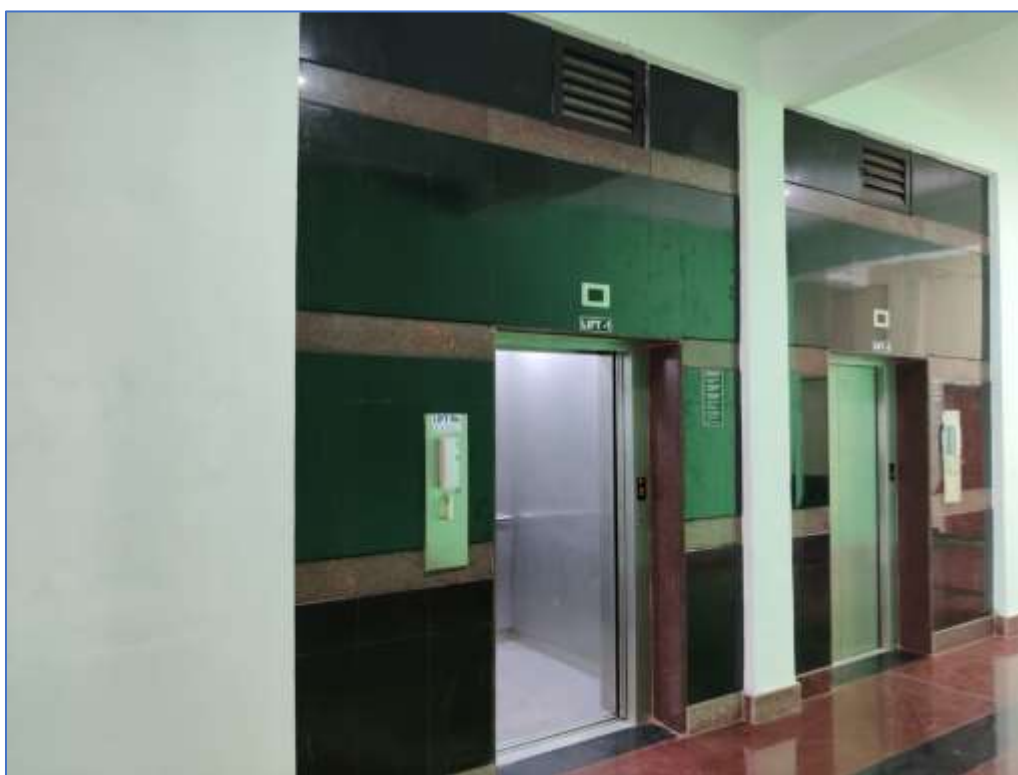
Lift – Administrative Block
