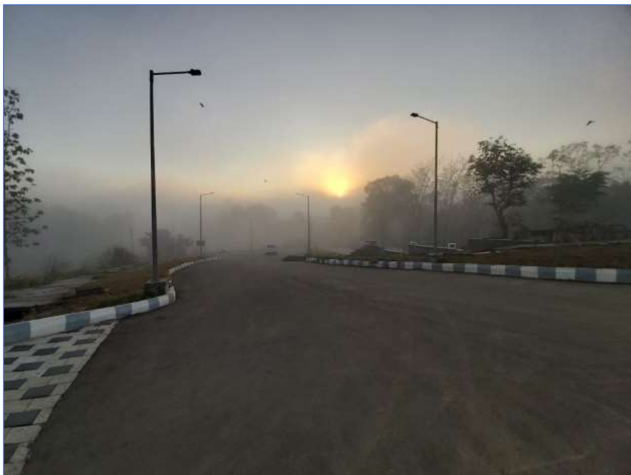
Roads inside the campus - Early Morning View
